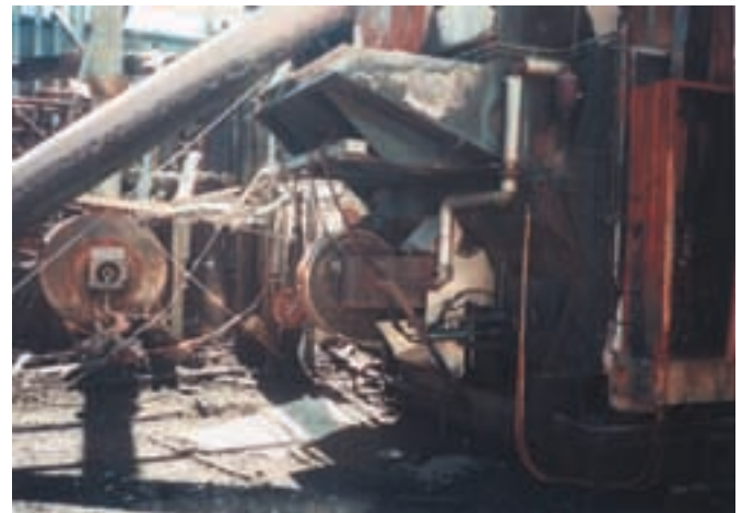
Aftermath of a boilerhouse fire
