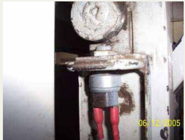
Gate cam and switch with missing plunger.
