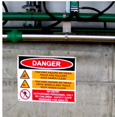
People in the pit to be alerted to possible risks.
