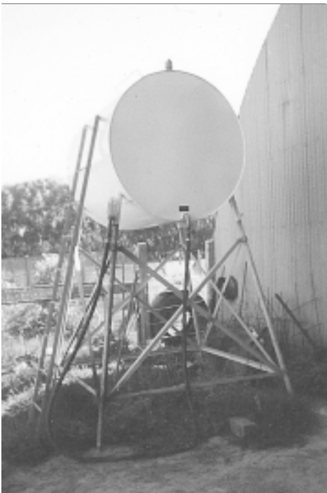
Where possible, locate petrol tanks in shade and have them painted in a light colour.
