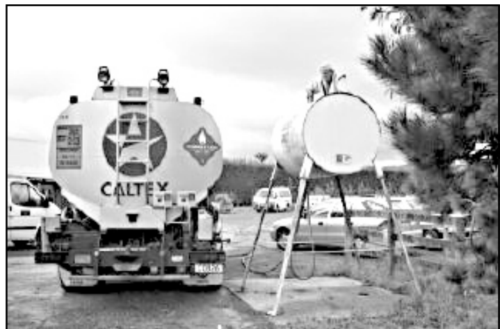
Preventing subsidence is best achieved by mounting the tank legs on a concrete pad.
