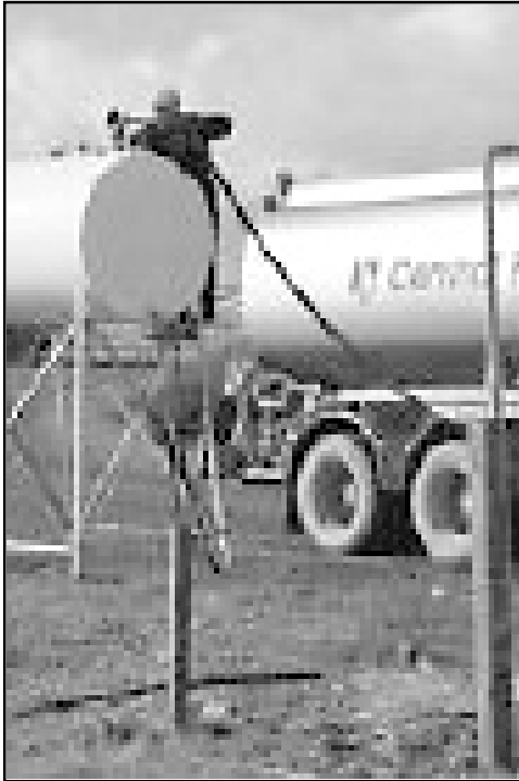
The area within 3 m of the tank shall be free of all obstacles.
